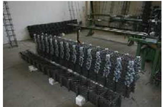
Plastbau eWall is uniquely characterized by being pre-reinforced with a steel ladder of size and spacing that automatically meet vertical reinforcement of the system. The vertical steel ladders, fitted with steel form ties, wedged by a stopper, and connected together by screw caps. The steel form ties are designed to form a regular grid points that are 20cm on centers and provides a seat for horizontal bars to be placed if desired.
