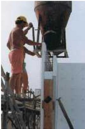
Concreting is done according to any requirements specific to a construction project and provisions such as ACI 301 and ACI 306 have addressed special precautions that need to be taken for structural and hot weather concrete respectively. Since the EPS form stay in place, concrete placed within the Plastbau eWall completely moist cured for the requisite 28 days. This makes it possible for the concrete to attain higher 28 days compressive strength by as much as 20 to 50%.
